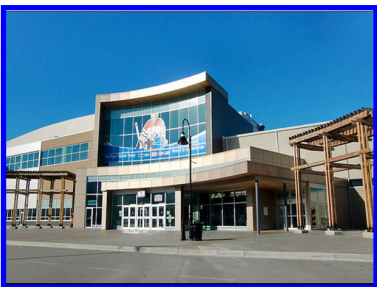
South Okanagan Events Center
